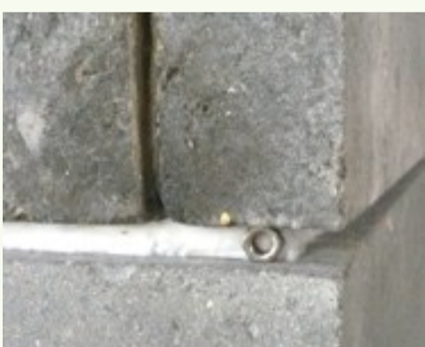
A nut can also serve as a spacer
