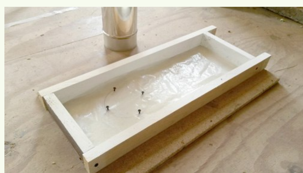
Exhaust block 550x200x50 mm with a Ø 122 mm opening for the flue pipe
